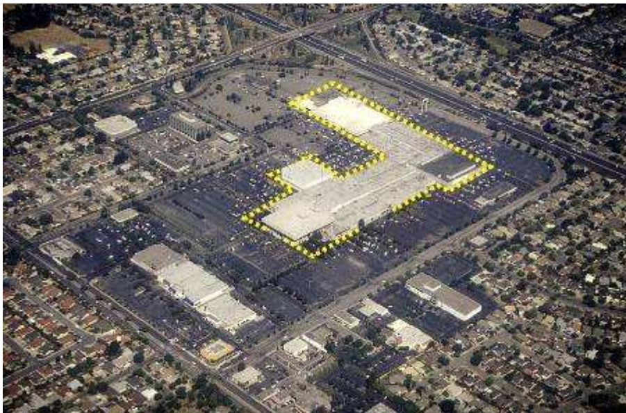
Enclosed private shopping centre - very high butt co-efficient
